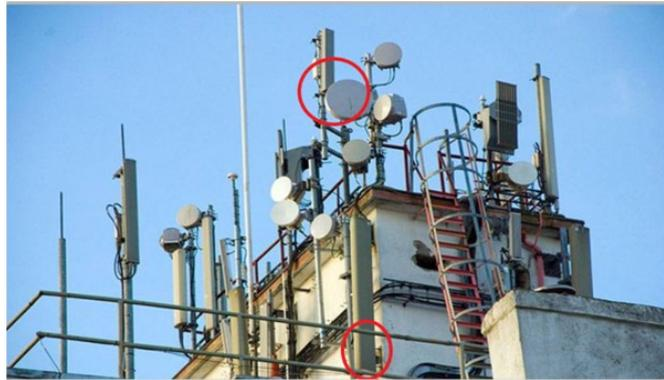
**2 – Physical effects.** If the antennas radiate into a PIM reflective material, for example, a rusty roof or rusty chain fence. With densification efforts ongoing it is increasingly difficult to find “clean” cell sites that are PIM free. Even tower mounted antennas commonly suffer from PIM due to the equipment mountings themselves. Rooftop sites inherently contain metal air-conditioning & plant equipment which can be common sources of PIM.
